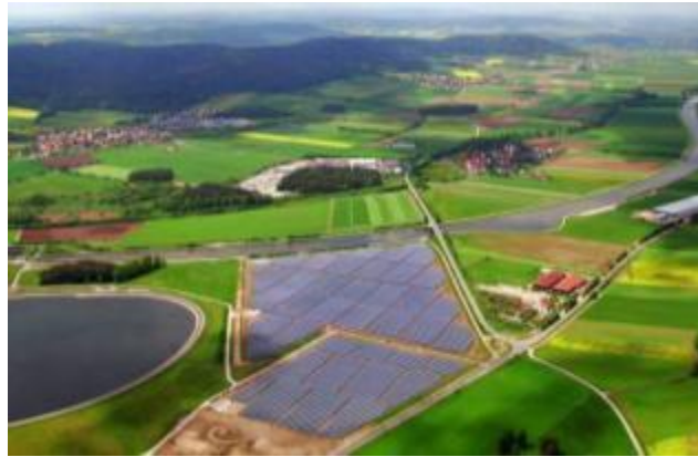
Muehlhausen, Bavaria, Germany, 6 MW SunPower T0 Tracker
