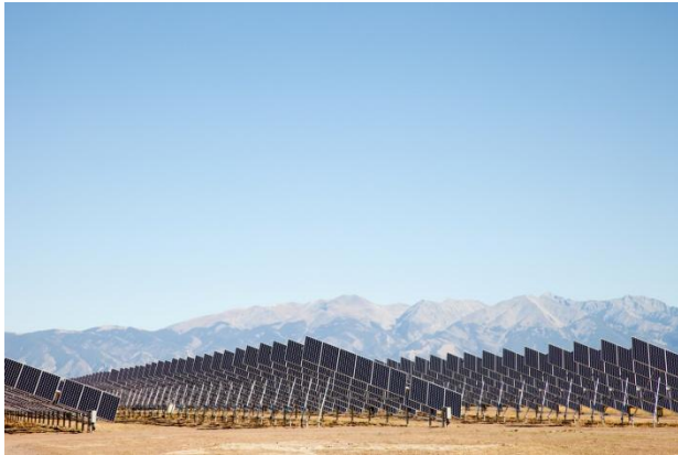
Greater Sandhill, Mosca, Colorado 19 MW SunPower T20 Tracker
