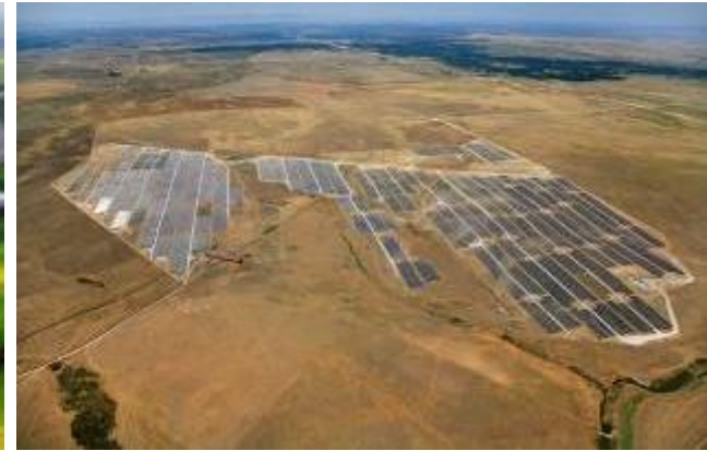
Trujillo, Extremadura, Spain-Elecnor 23 MW SunPower T0 Tracker
