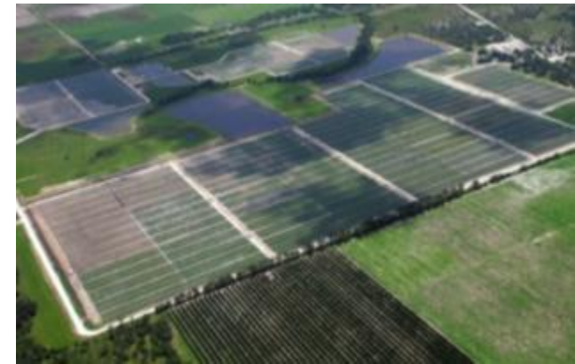
DeSoto, Arcadia, Florida 25 MW SunPower T0 Tracker
